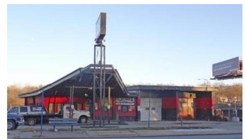
Phillips Service Station - Willy's Petroleum Co. 5901 Prospect Ave. Photos by KCModern Survey
