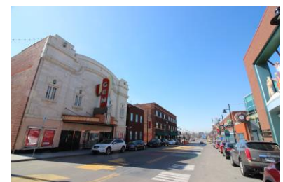
18 th and Vine Historic District looking West
