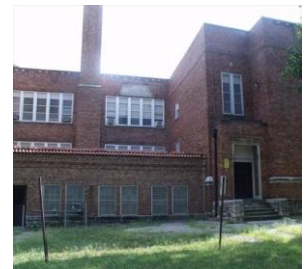
Pershing School, 5915 Park Ave
